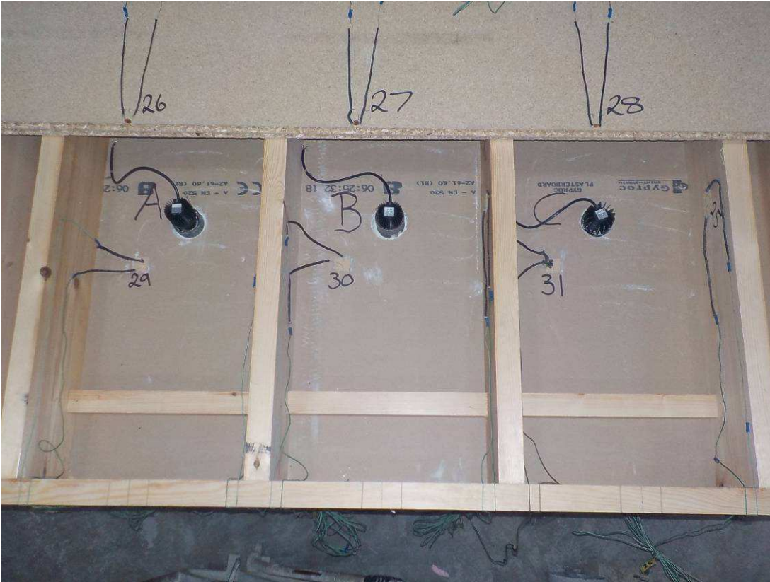
Photo 2.1.9 – Downlights A,B and C
