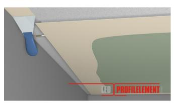
17. Fill all adjoining profile edges and screw fixings.
