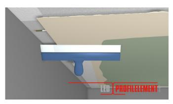
Once the fleece is dry, trim any that protrudes over the edged. Fill the fleece strip with standard filler.
