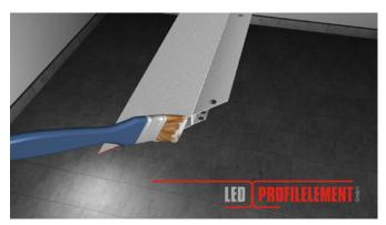
**03.** File or sand cut edges. Re-apply primer to the cut edges (e.g. standard zinc primer).
