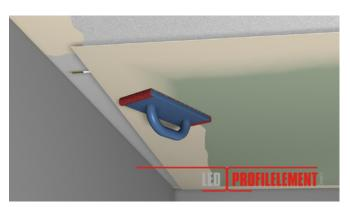
23. Sand back the filled profiles and surfaces. Avoid leaving an uneven surface that may break the light. Surface quality Q3 or Q4.
